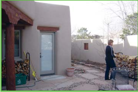
Move firewood away from structures.
